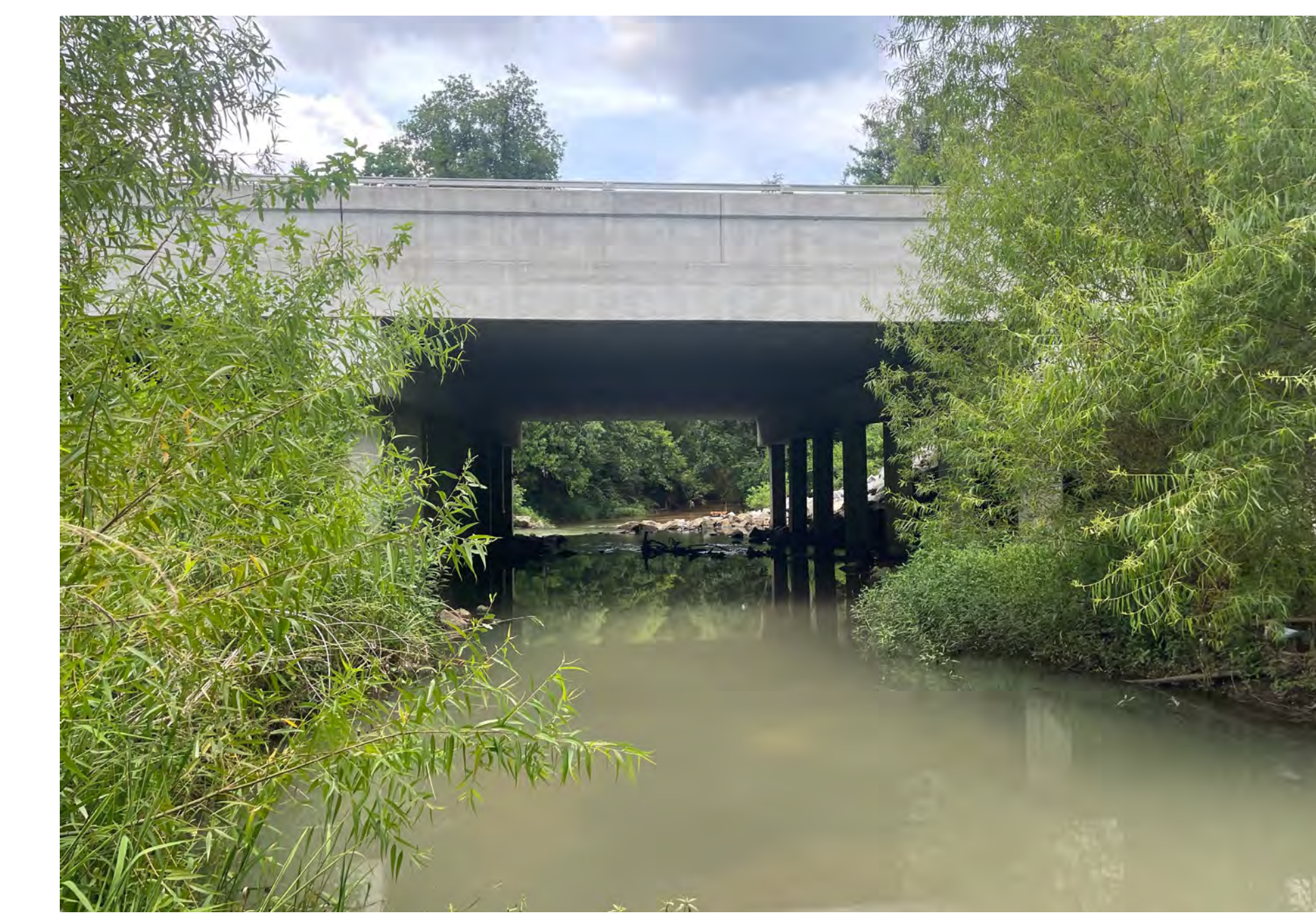
4 As seen from the N 9th Ave crossing, the creek appears polluted, trash littered along the edges.
