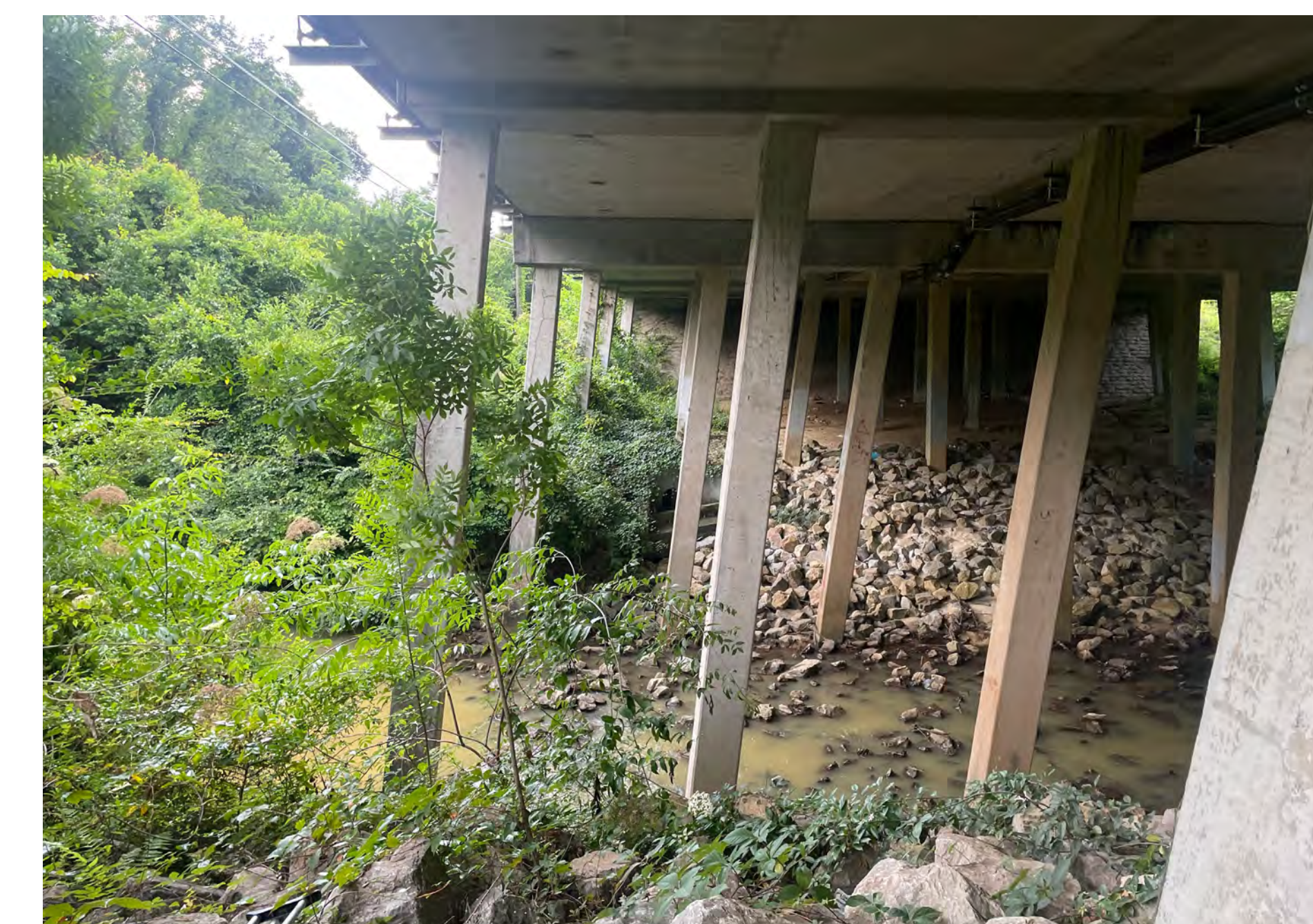
3 Carpenter Creek underneath Airport Blvd bridge, termination of concrete slough alongside crossing. Likely the highest clearance of crossings.
